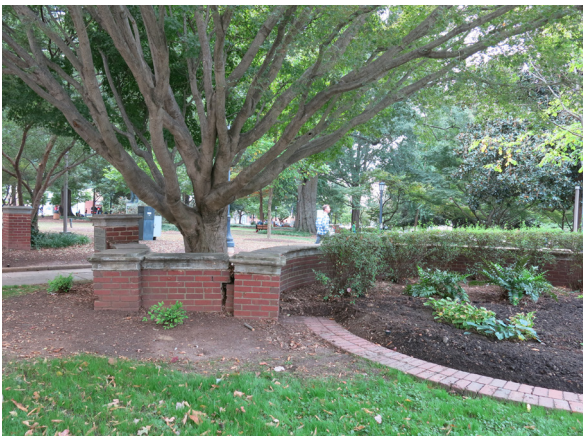
Corner brick walls (1940/1954) with contemporary planting beds (RATIO)
