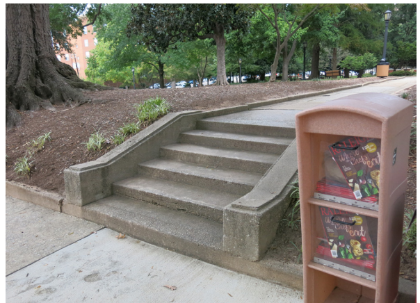
Concrete steps and walkway (c.1940) (RATIO)
